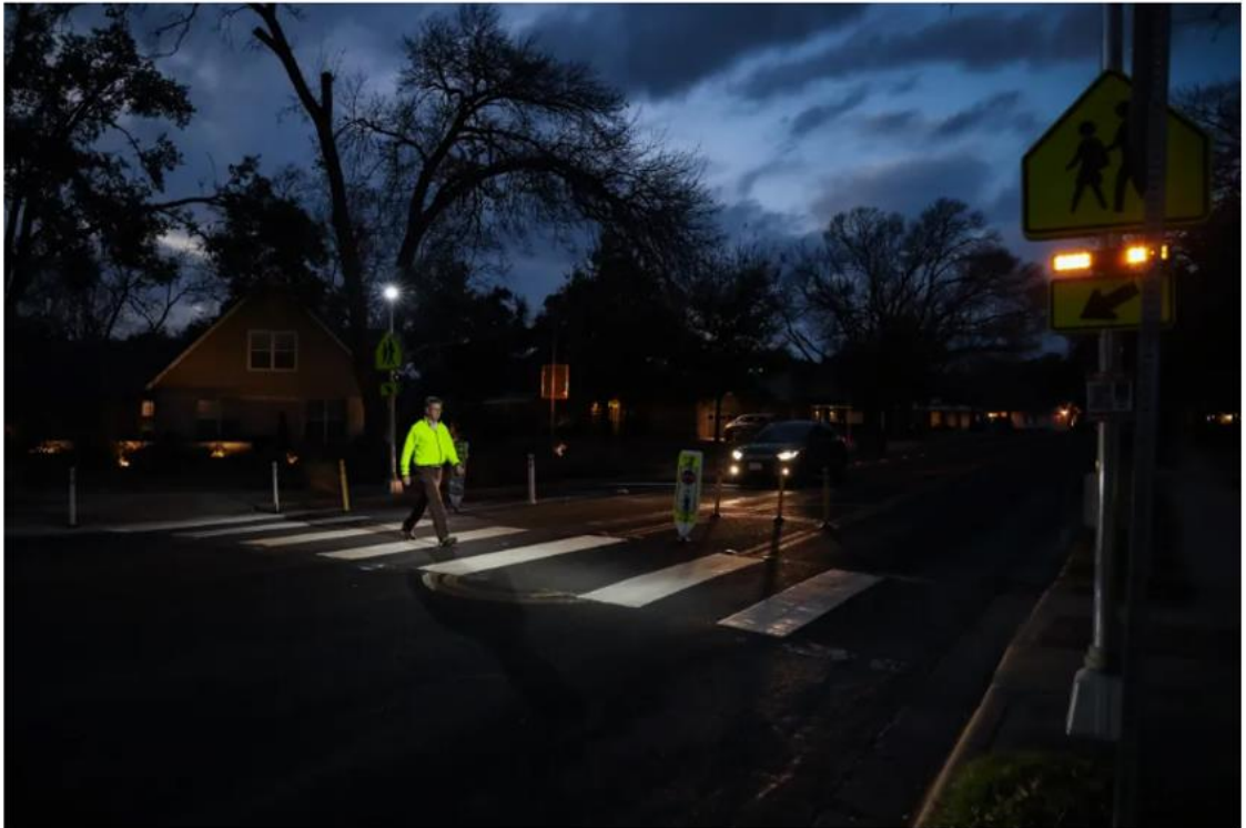
Figure 22 Austin—Solar-Powered Flood Lights on RRFB
